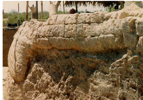
Fig. 24. The edge of the lower wall of the Lagumbyee kiln is rounded where the unhardened section of the large raw clay bricks later eroded.
