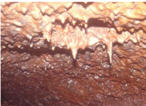
Fig. 11. Inground kiln ceiling eroded by fusion (melting). Sawankhalok (Thailand).
