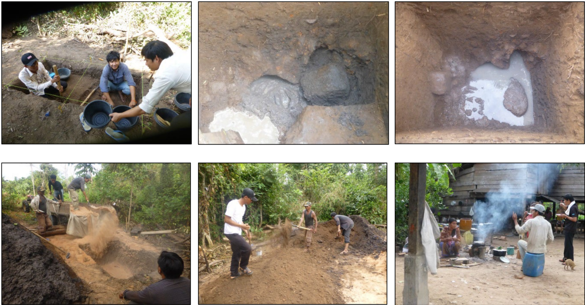
Figs. 3-6. Suite of images showing the progress of the November 2014 excavation, including the team beginning the dig; the laterite block in front of the righthand stokehole; the intrusion of ground water; backfilling with sand and 'making good' with top soil; and a moment of rest at the conclusion of the work.
